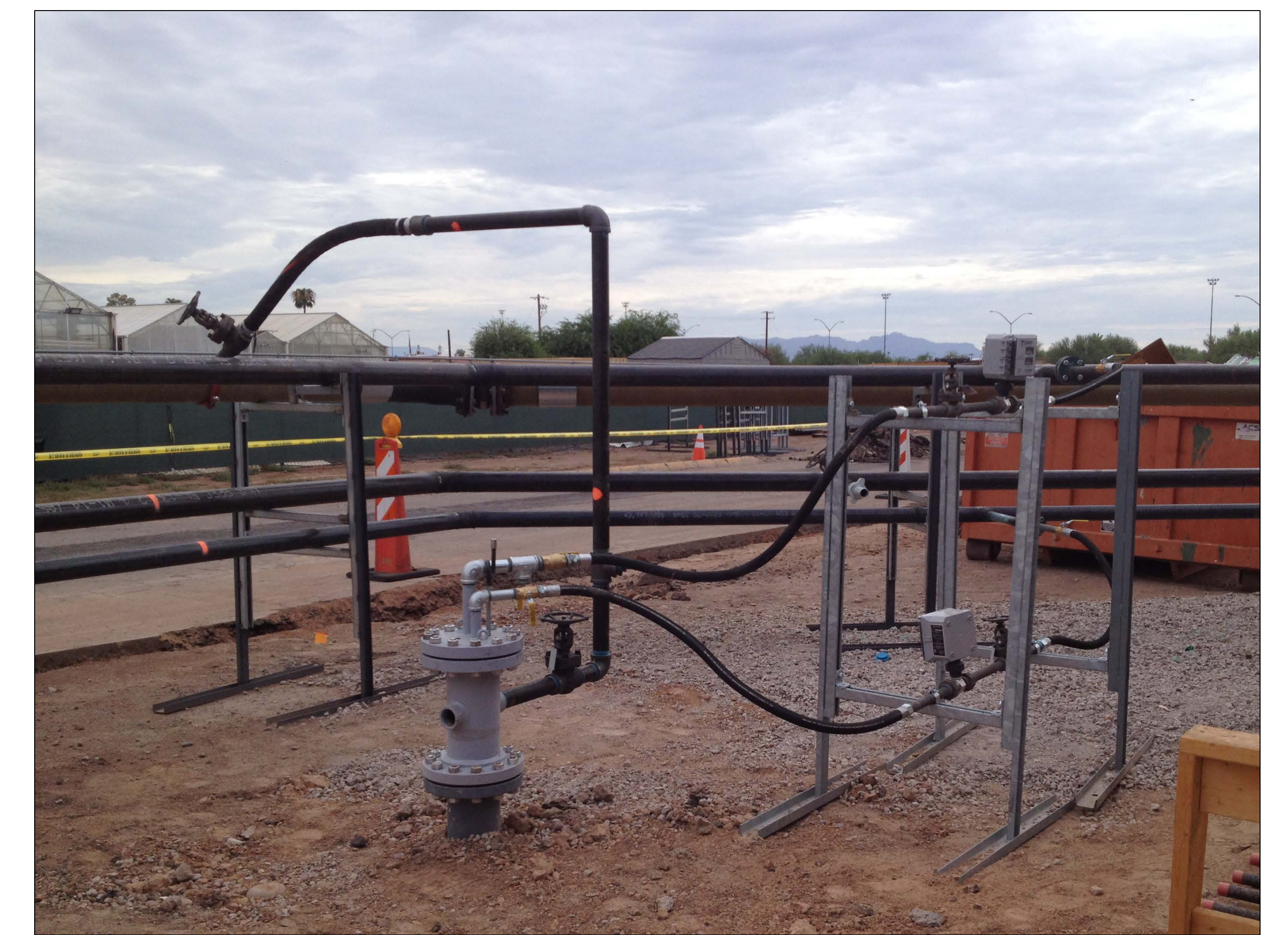
Multi-Phase Extraction Well
