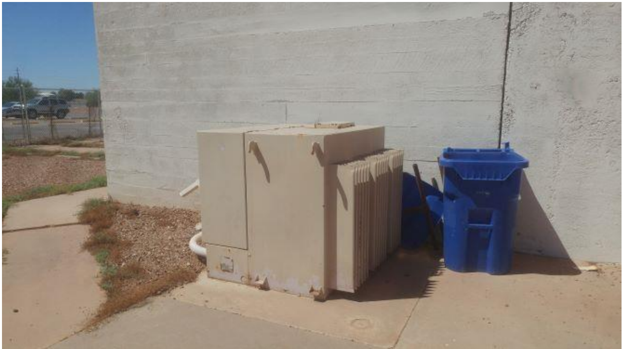
Photo 2: Transformer at Building 715, September 6, 2018, view West
