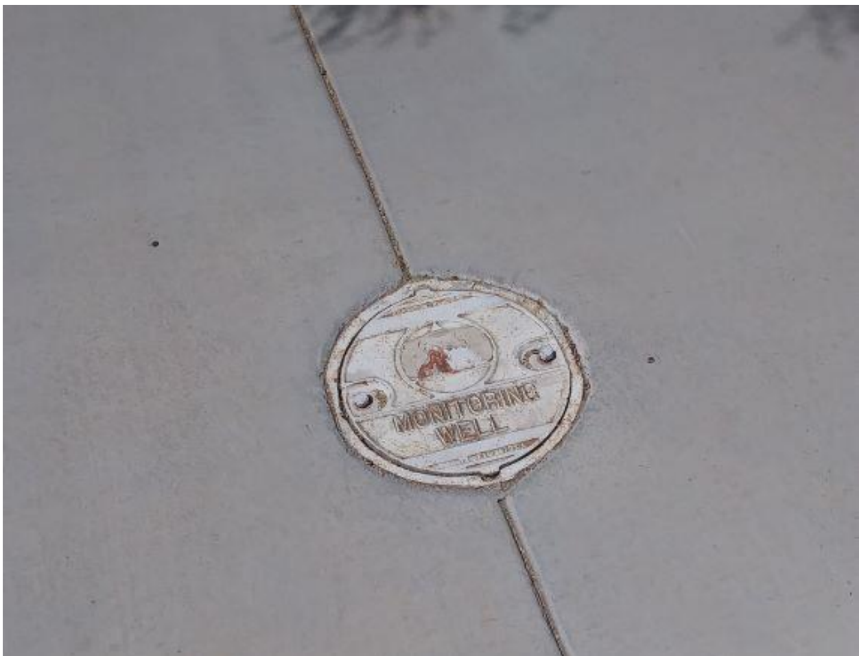
Photo 12: Flush mounted monitoring well (typical of two), outside fence on east side of Parcel, September 6, 2018, view South
