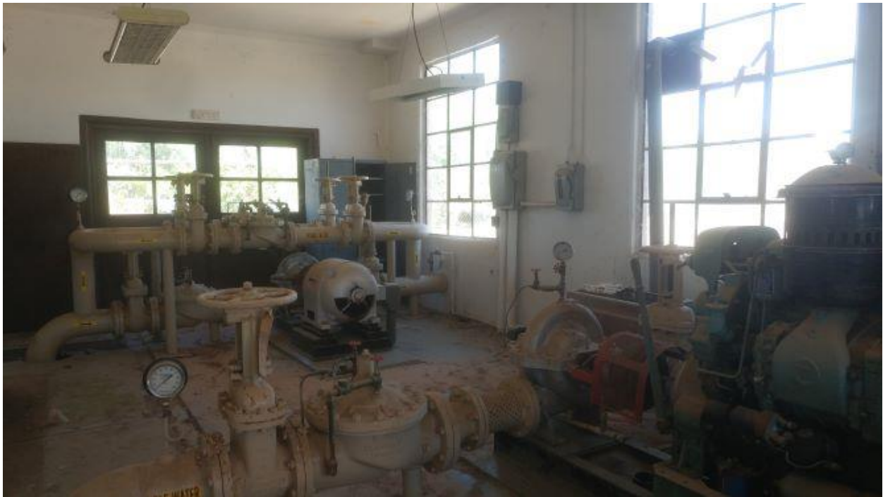
Photo 3: Building 715 Pump Room, September 6, 2018, view North
