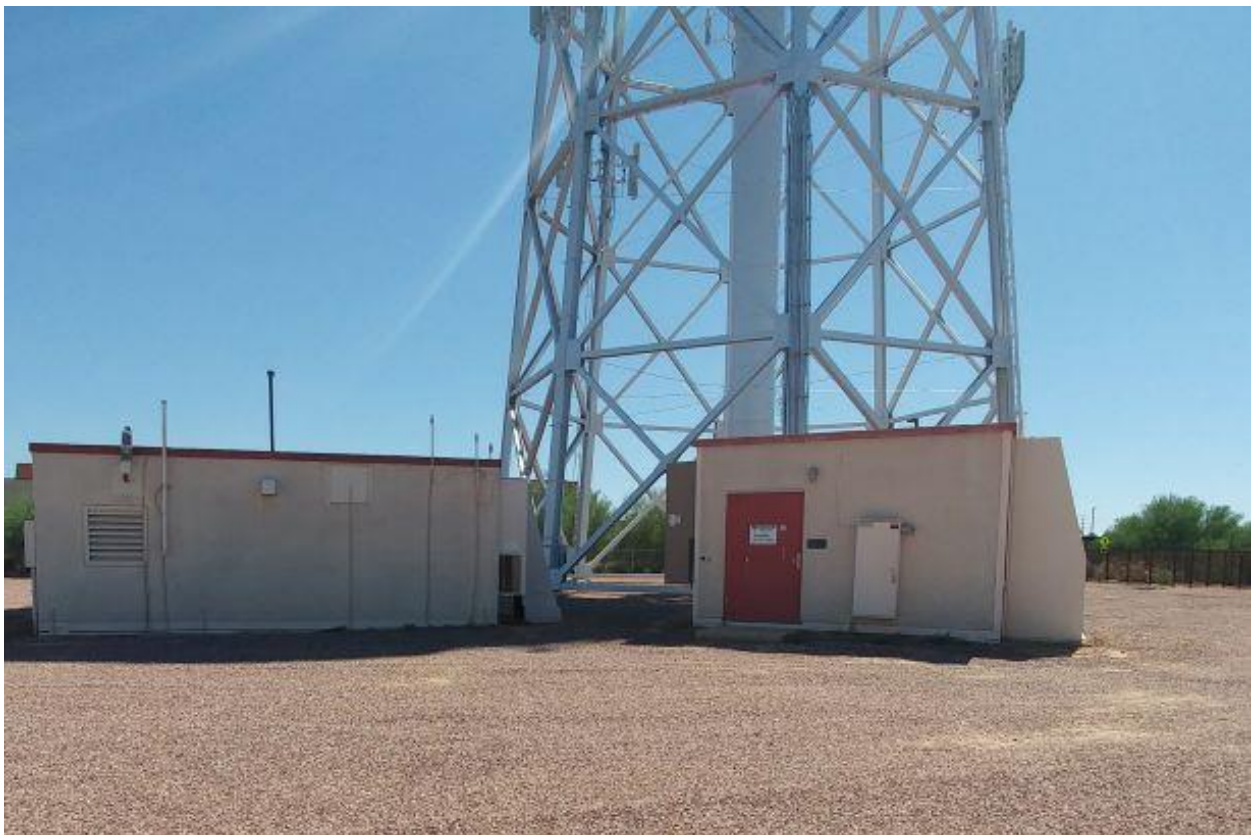
Photo 10: Telecommunication buildings, September 6, 2018, view East
