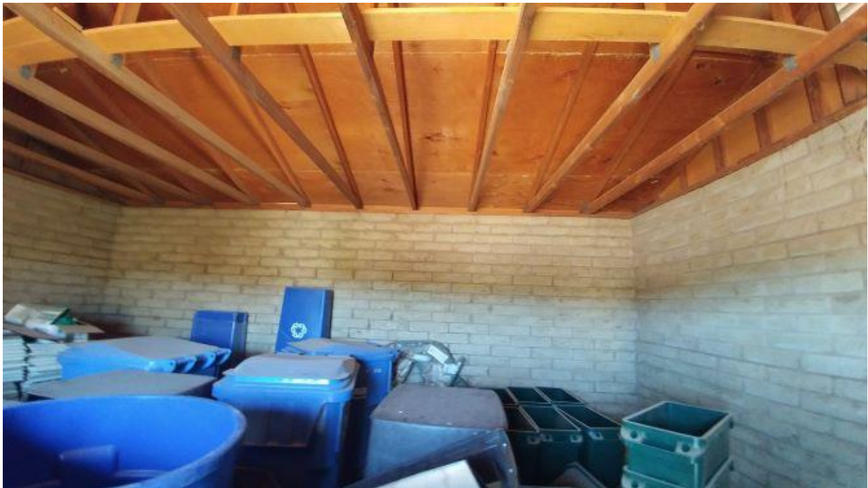
Photo 8: Inside Building 716, September 6, 2018, view West
