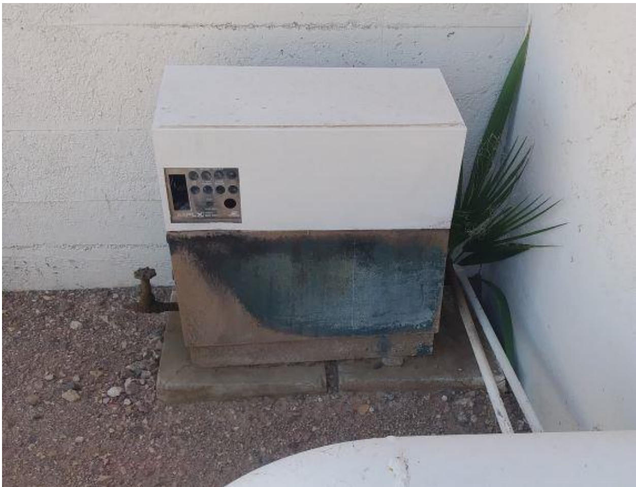
Photo 6: Building 715 diesel day tank on west side, September 6, 2018, view East
