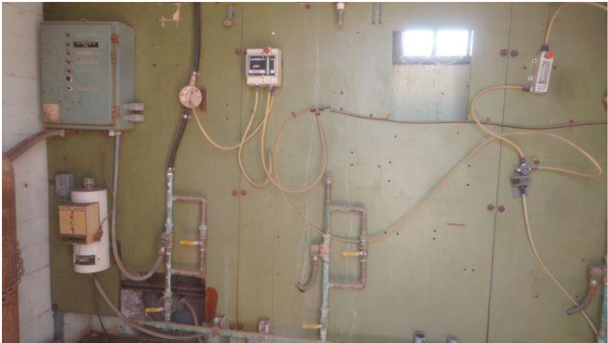
Photo 5: Building 715 chemical mixing room, September 6, 2018, view West
