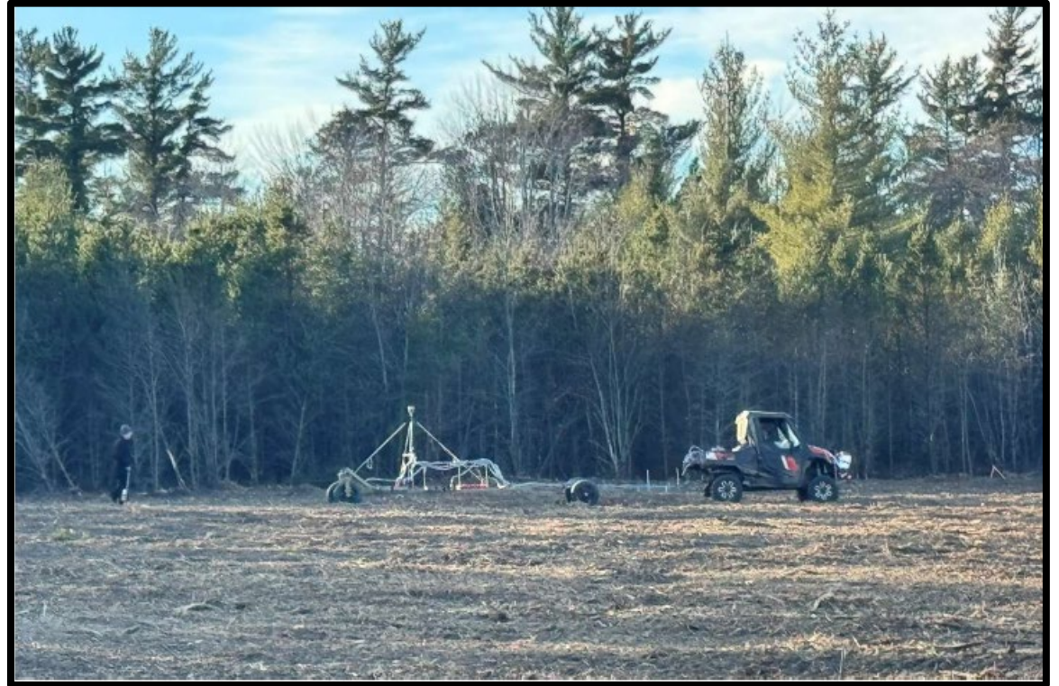
Work team mobilized to the site Oct 2, 2025, to begin clearing activities
