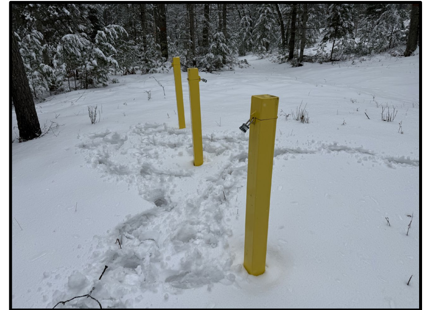
Groundwater monitoring wells in winter
