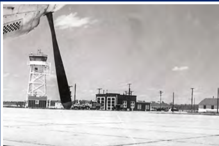
England Air Force Base Control Tower, circa 1953
