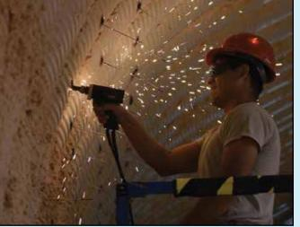
Senior Airman Daniel Torres, a member of the 819th RED HORSE Squadron structures shop, performs pin welding to install new insulation on a storage facility at Malmstrom Air Force Base, Montana, May 20, 2015. The 819th RHS provides heavy repair capability and construction support when requirements exceed normal base civil engineer capabilities and where Army engineer support isn't readily available. (U.S. Air Force photo/Chris Willis/Released)
