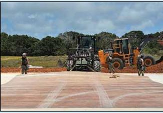
Air Force civil engineers pull folding fiberglass matting over a crushed stone crater repair during a Silver Flag airfield damage repair exercise at the Pacific Regional Training Center on Northwest Field, Guam. (U.S. Air Force photo/Airman 1st Class Emily A. Bradley/Released)
