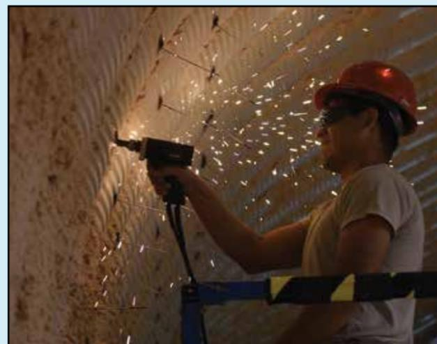
Senior Airman Daniel Torres, a member of the 819th RED HORSE Squadron structures shop, performs pin welding to install new insulation on a storage facility at Malmstrom Air Force Base, Montana, May 20, 2015. The 819th RHS provides heavy repair capability and construction support when requirements exceed normal base civil engineer capabilities and where Army engineer support isn't readily available. (U.S. Air Force photo/Chris Willis/Released)
