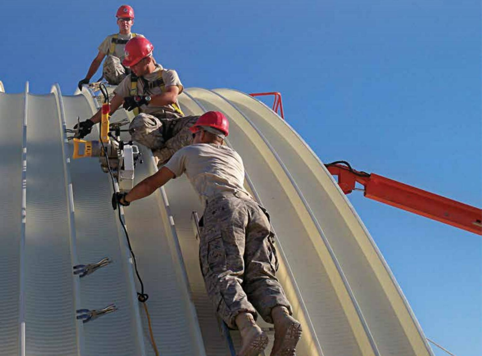
(facing page) Civil Engineers from the 820th RED HORSE Squadron work to seal a K-Span at an unknown location. (U.S. Air Force photo/ Mark Hanley/Released)
