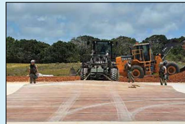
Air Force civil engineers pull folding fiberglass matting over a crushed stone crater repair during a Silver Flag airfield damage repair exercise at the Pacific Regional Training Center on Northwest Field, Guam. (U.S. Air Force photo/Airman 1st Class Emily A. Bradley/Released)
