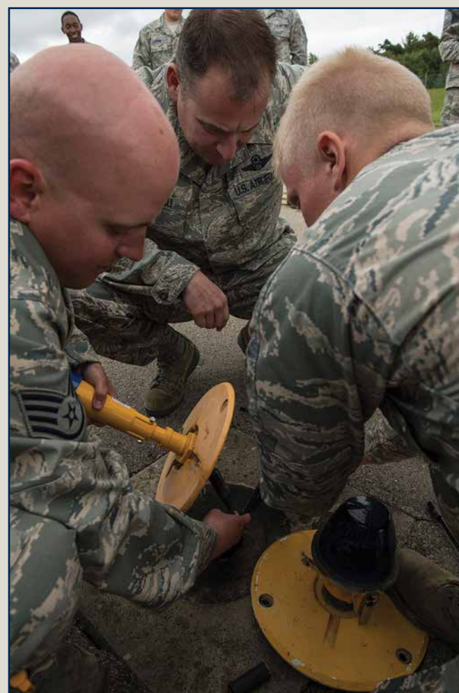
Taxiway Tuesdays, a previous contest entry, led to the replacement of traditional taxiway lights with light-emitting diodes. The project is saving 400 man-hours and uses 75 percent less power annually. (U.S. Air Force photo/Staff Sgt. Christopher Ruano)
