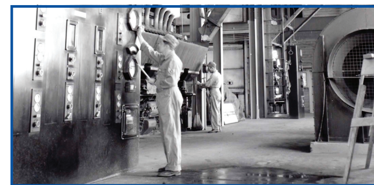
Air Force civil engineers check the gauges at a utility plant in the 1960s.
