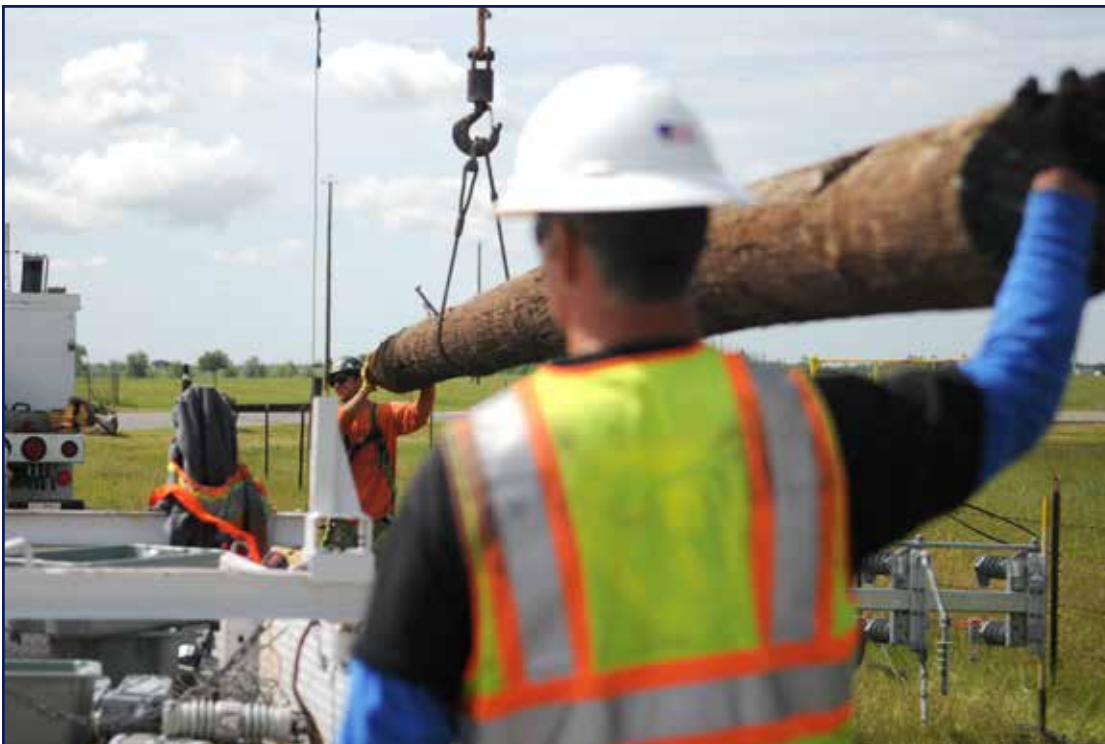
Workers load a power pole onto a truck to make room for its replacement at Beale Air Force Base, California, April 24, 2017. The new poles will be able to supply Beale’s increased energy demands in addition to weathering storms more reliably. (U.S. Air Force photo by Airman 1st Class Douglas Lorange)
