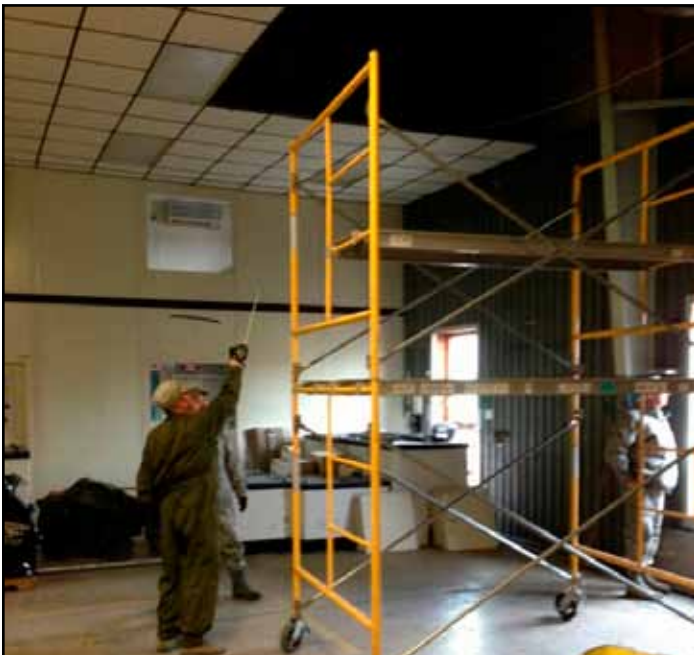
Installation of ceiling tiles during renovation
