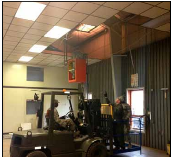
Installation of lighting fixtures
