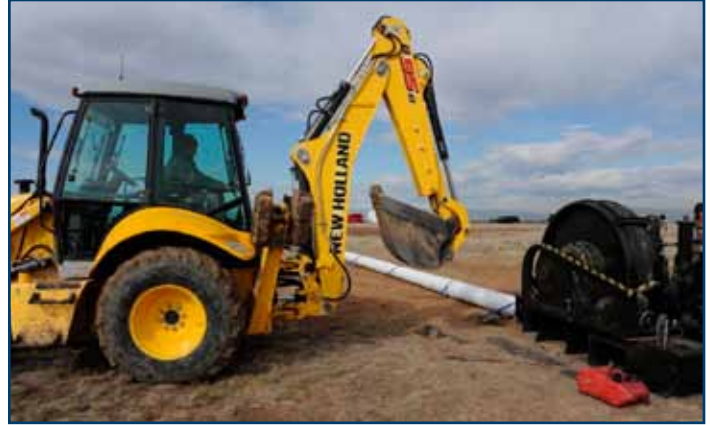
Team Member prepares to move BAK-12 into position during installation
